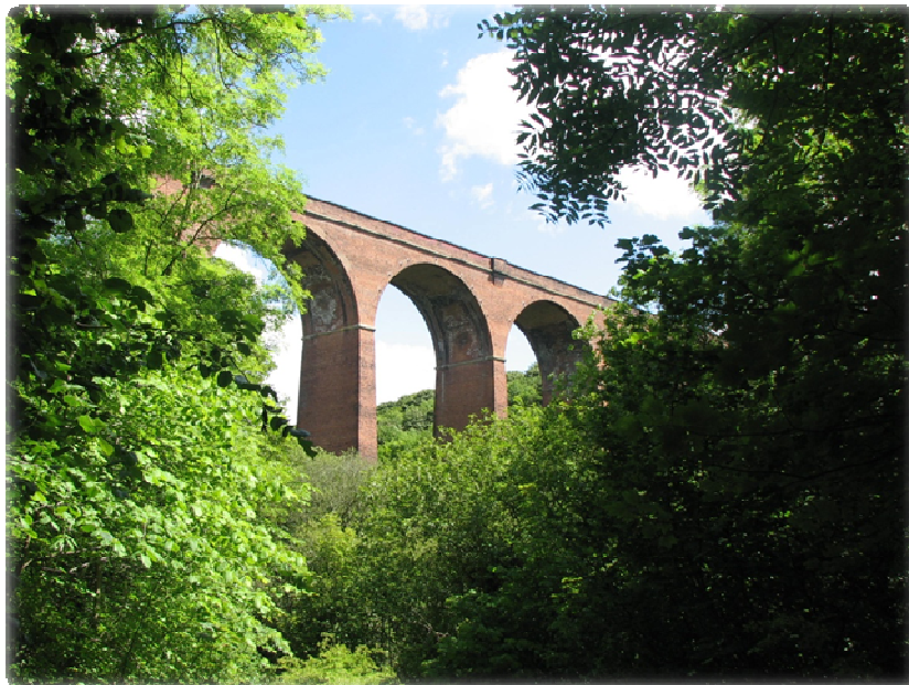
Crimdon Viaduct Photograph courtesy of Stan Gray
